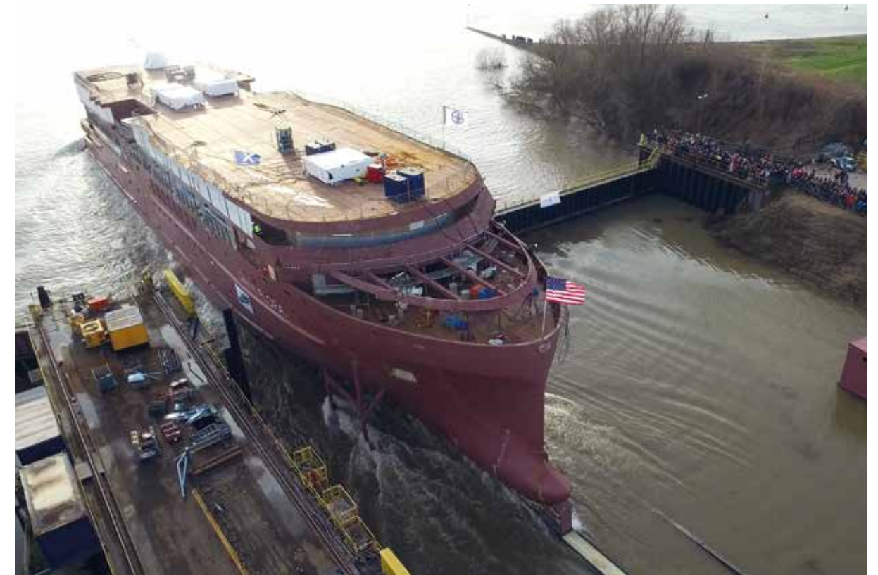
A building process of one and a half years on De Hoop's longitudinal slipway
