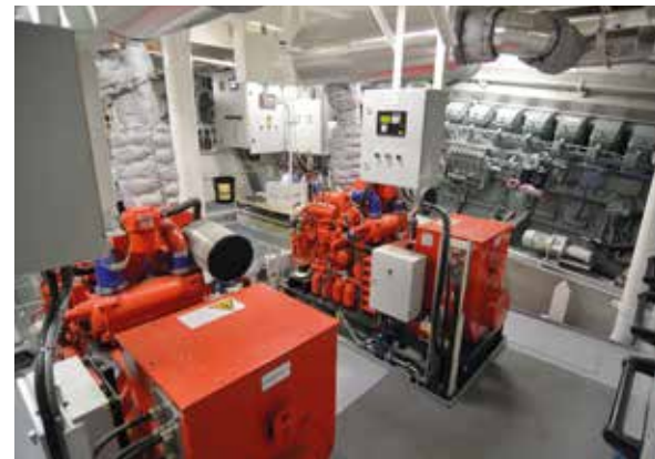
Two 116kW generator assemblies supply electrical power for the vessel
