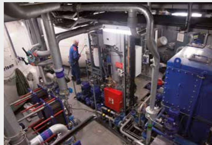
Two of the four dry bulk tanks and the sewage tank in the fore ship below the superstructure
