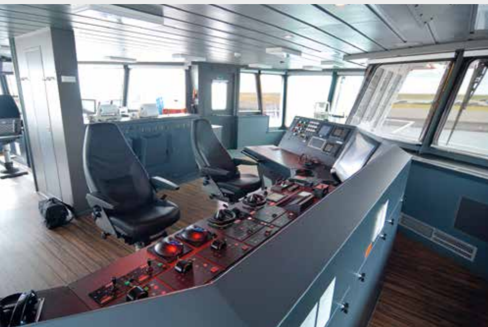
The bridge comprises an extensive package of nautical, navigation and communication equipment
