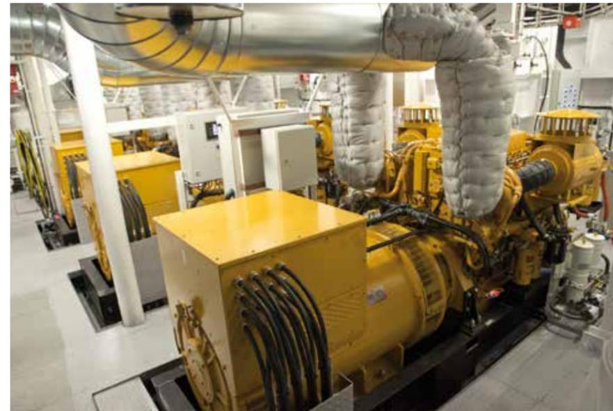
Power generation comprises of four diesel alternators of 995 kW each
